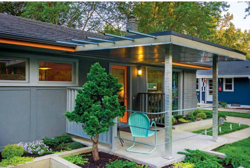
TWO SHINY ALUMINUM POSTS ARE JOINED BY EXTRUDED METAL TUBING AS A RAILING ON THE NEW PORCH. THE CEILING PANELS, A SANDWICH OF TWO LAYERS OF ALUMINUM OVER PVC, VIRTUALLY DISAPPEAR ABOVE THE POURED CONCRETE FLOOR. "THE ORIGINAL PORCH ALSO HAD TWO PARTIAL LOUVERED WALLS; WE INCLUDED UPDATED VERSIONS OF THOSE, ADDING BOTH TO THE PRIVACY AND THE DESIGN AESTHETIC," ELIN SHARES.
