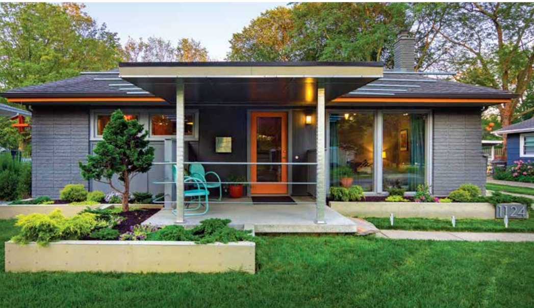
TWO SHINY ALUMINUM POSTS ARE JOINED BY EXTRUDED METAL TUBING AS A RAILING ON THE NEW PORCH. THE CEILING PANELS, A SANDWICH OF TWO LAYERS OF ALUMINUM OVER PVC, VIRTUALLY DISAPPEAR ABOVE THE POURED CONCRETE FLOOR. "THE ORIGINAL PORCH ALSO HAD TWO PARTIAL LOUVERED WALLS; WE INCLUDED UPDATED VERSIONS OF THOSE, ADDING BOTH TO THE PRIVACY AND THE DESIGN AESTHETIC," ELIN SHARES.
